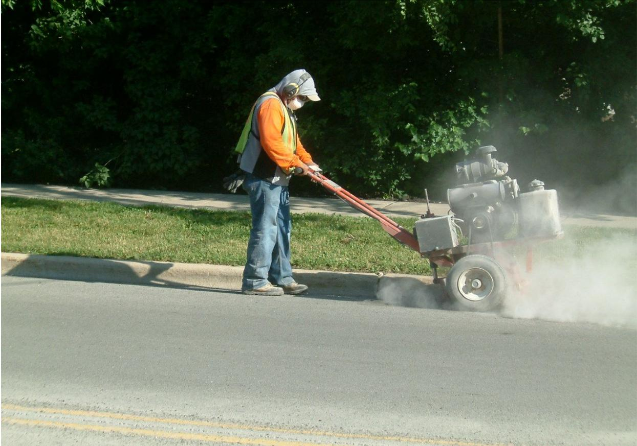
TK Sealcoating of St. Charles IL performs Parking lot Crack Sealing which is one of the most important maintenance events for asphalt parking lots and all pavement surfaces. Hot rubber or liquified rubber is used to seal the cracks in the pavement and prevents and slows water from destroying the stone base and subbase of your parking lot or roadway. The goal is to seal the cracks so that the water runs off the pavement and does not erode the base or foundation of pavement.
